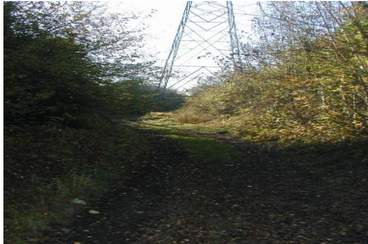
ESB pylon to be relocated
