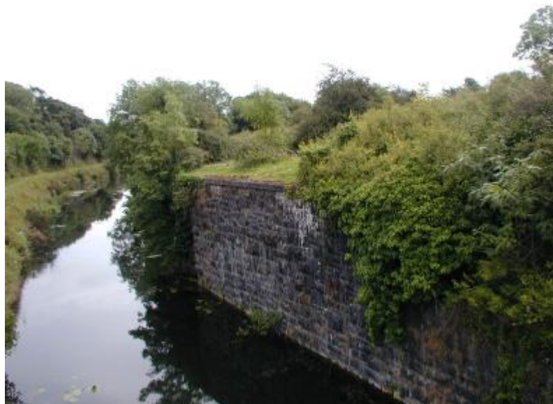
Existing bridge abutments at Royal Canal
