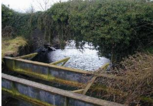
Bridge over river at Bennetstown
